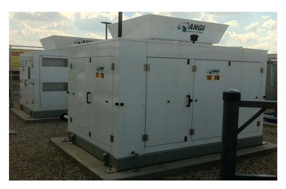
Typical CNG compressor packages, courtesy of ANGI Energy Company
